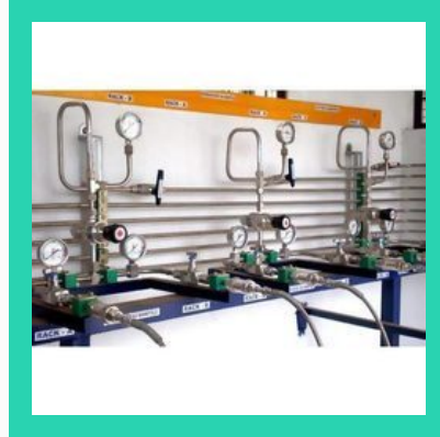
Co2 Gas Pipe Line Work
